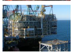
Scope of Work: Our SOW included the construction engineering, partial procurement, fabrication, mechanical completion, commissioning assistance and load-out of the Production deck with a total weight of 10,500 tons. The Production Deck consists of an integrated, single lift structure, 60m long x 24m wide over main truss lines, and 26m high, top of cellar deck to top of weather deck.
