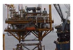
Project Specifics: The modernization works included the addition of new structural facilities, control systems and Fire & Gas systems, Emergency Shut down, Power Generation and Distribution, Gas Compression, Plant and Instrument Air Systems, Lighting and Small Powers, Life Safety Systems, Gas Combustible, ad HVAC.
